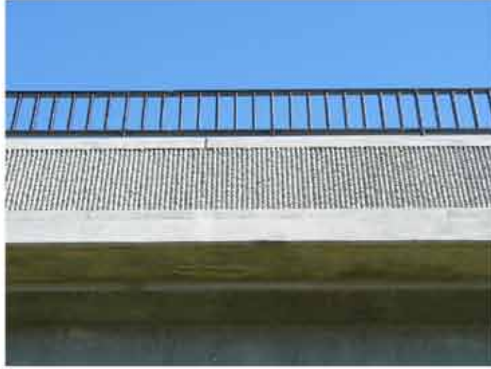
Fractured-fin formed concrete parapet with pedestrian railing
