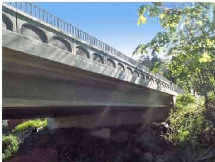
Filled-arch concrete parapet with pedestrian railing
