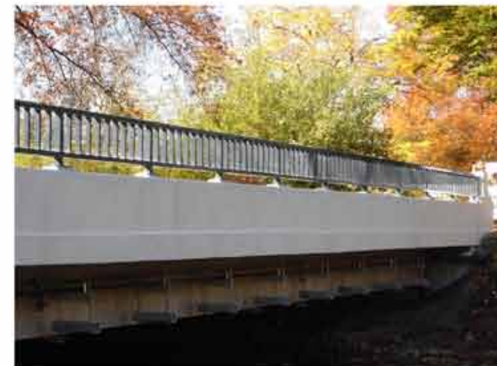
Plain finished concrete parapet with pedestrian railing
