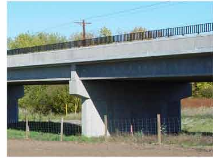
Concrete pier wall
