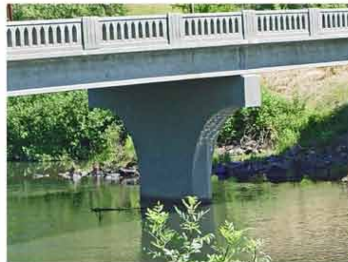
Flaired top concrete pier with diamond shaped ends
