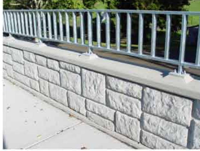
Ashlar stone formed concrete parapet with pedestrian railing
