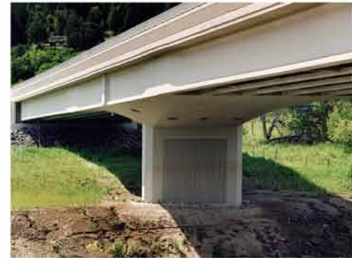
Diamond shaped concrete pier with fractured-fin treatment
