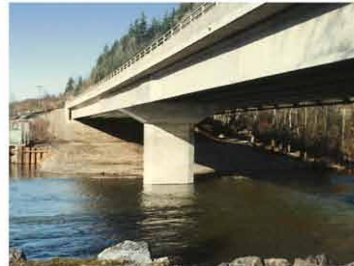
Diamond shaped concrete pier with smooth finish
