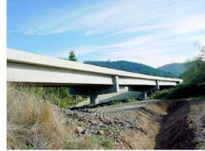
Concrete Type F railing
