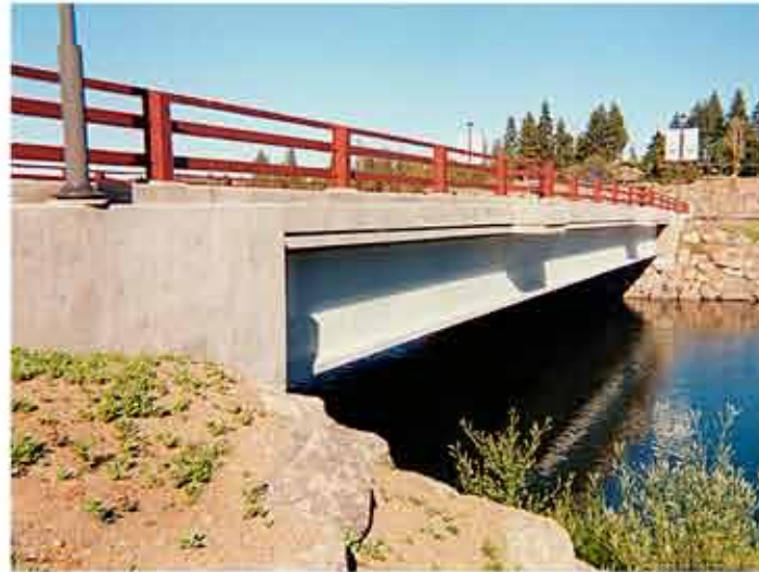
Three-tube curb-mount steel railing
