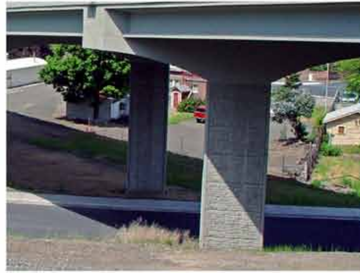
Ashlar stone formed concrete columns
