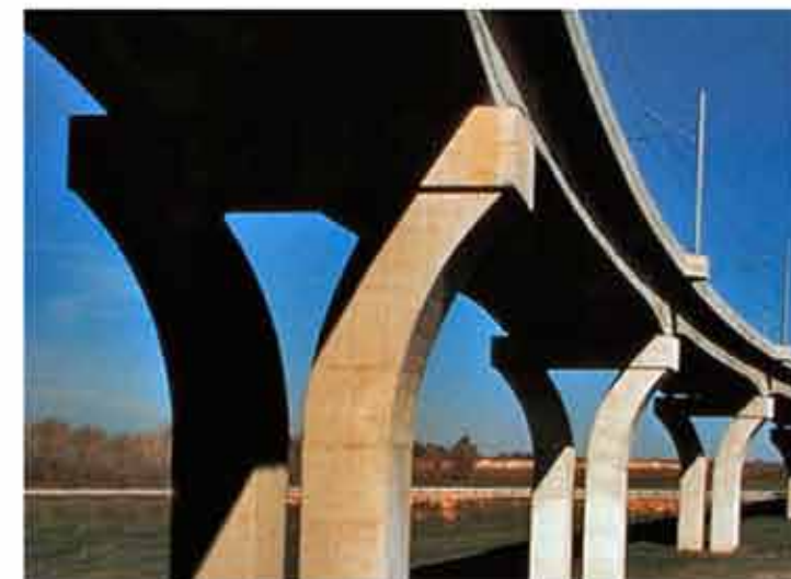
Y shaped concrete piers
