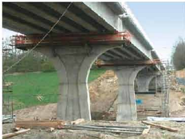
Flaired top concrete pier with recessed shape
