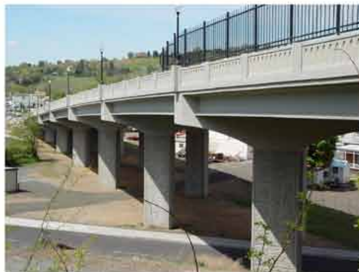
Concrete Texas-style railing with filled windows
