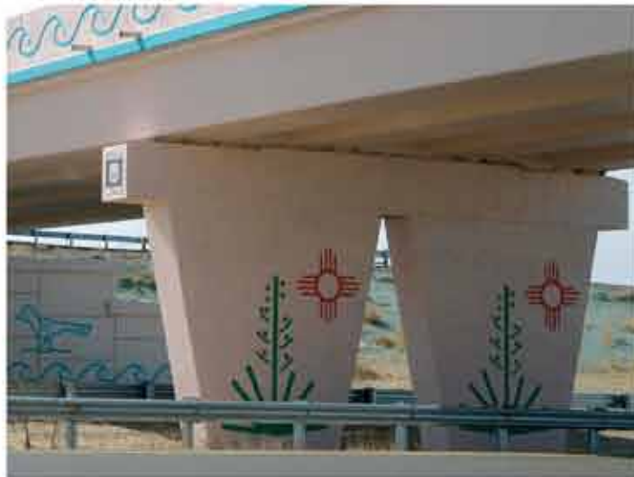
Decorated concrete tapered piers
