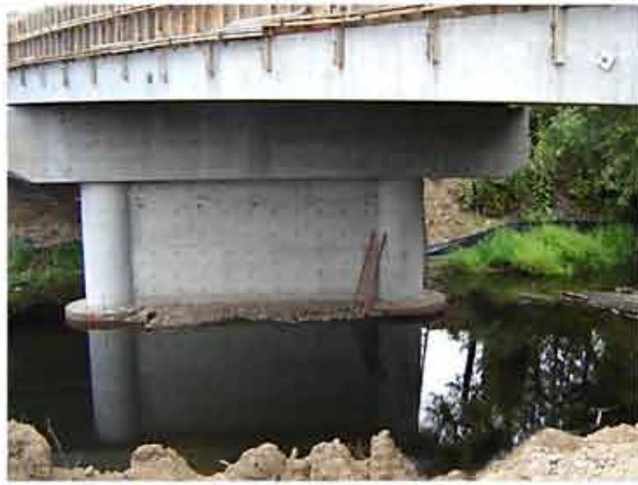
Round concrete columns with wall
